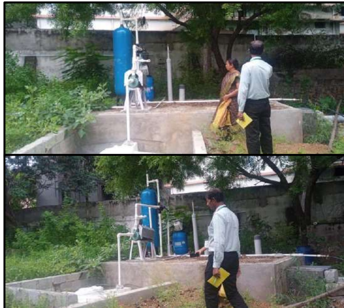
Waste Management Measures – Dustbins & STP units facilities observed at the Campus
